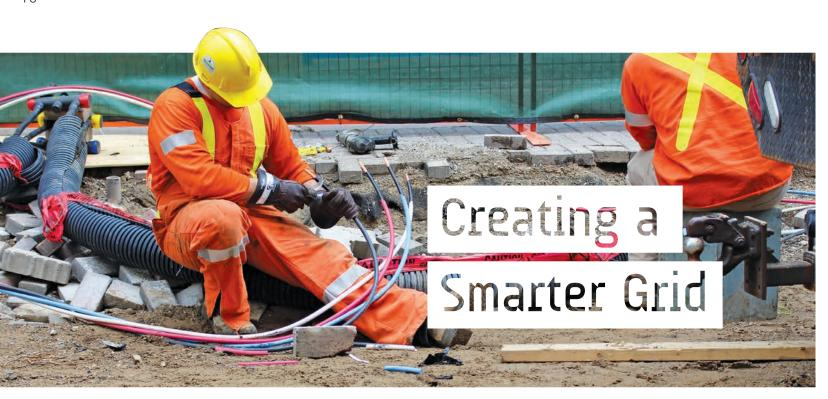
In 2017 London Hydro continued upgrading much of London's underground infrastructure in the City core. Duct systems, maintenance manholes, and cables are being replaced with a modern automated system including major work on Dundas Street in support of the Dundas Place Flex Street project.
