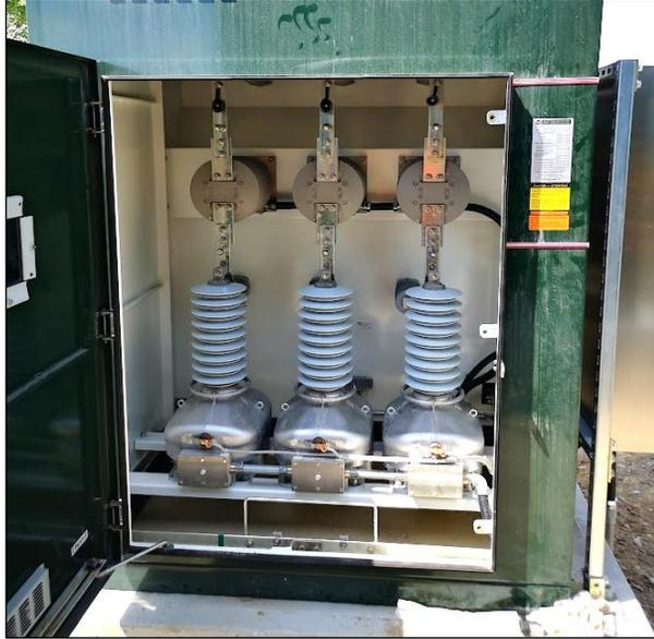
**Figure 3-7, Typical Primary Metering Unit**
