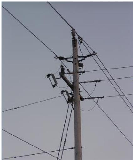
Figure 3-1, Typical Fused Tap Framing
