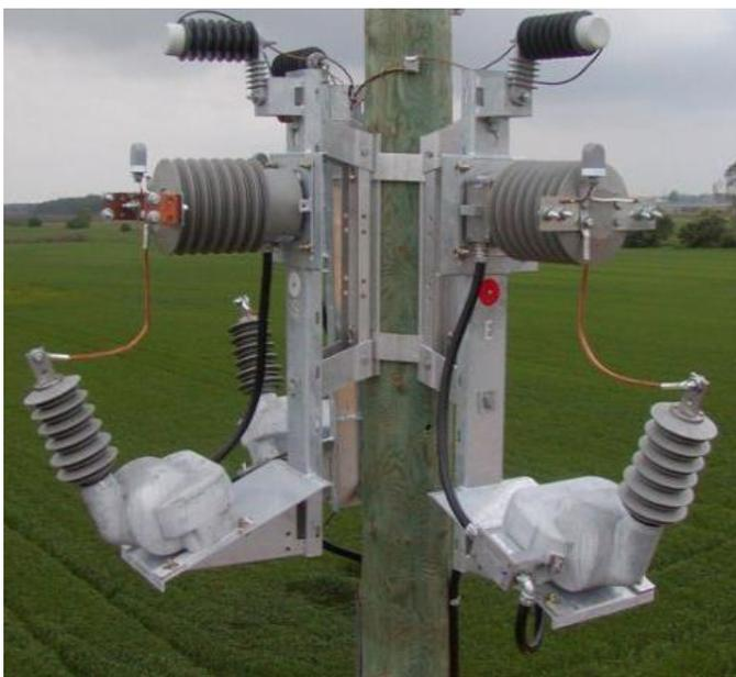
**Figure 6-1, Typical Primary Metering Unit**
