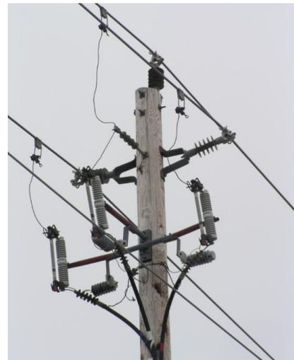
Figure 3-2, Typical Fused Riser Framing
