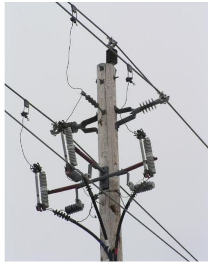
Figure 3-2, Typical Fused Riser Framing
