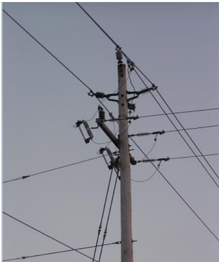
Figure 3-1, Typical Fused Tap Framing
